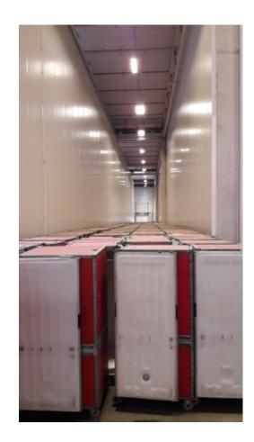
Before transport, isothermal containers designed to transport heat sensitive products are subjected to pre-cooling in the refrigerated area with a temperature of around 8  $^{\circ}$ C.
